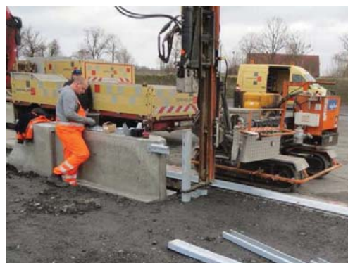
4.12 Rammen der Pfosten Driving in the posts
