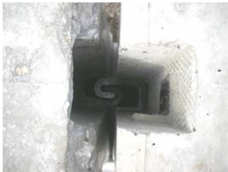
4.5 JJ-Hooks Krallenverbindung... JJ-Hooks connection...
