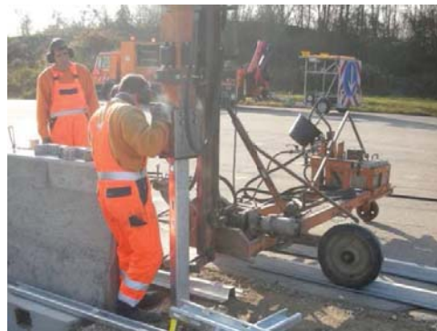
4.13 Rammen der Pfosten Driving in the posts
