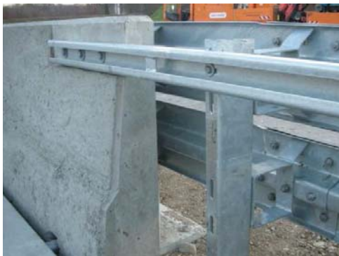
4.18 Anbindung des hinteren C-100 an das Betonwandelement Connecting the rear C-100 profile with the concrete wall element
