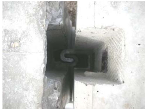
4.6 JJ-Hooks Krallenverbindung JJ-Hooks connection
