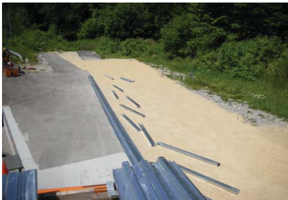
5. Laying outposts and brackets
