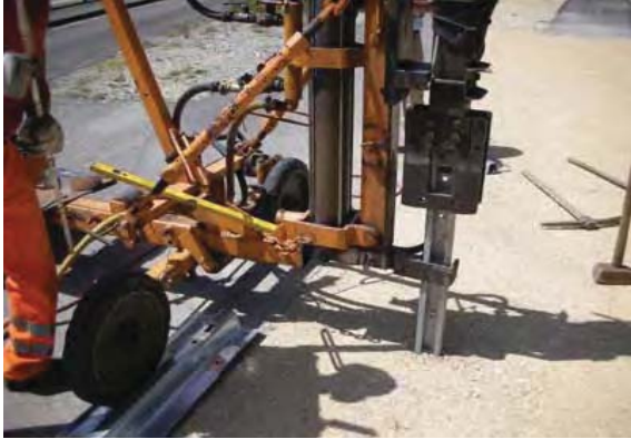
7. Driving posts into ground
