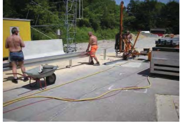
8. Pre Mounting brackets and beams
