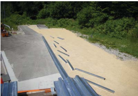
5. Laying outposts and brackets
