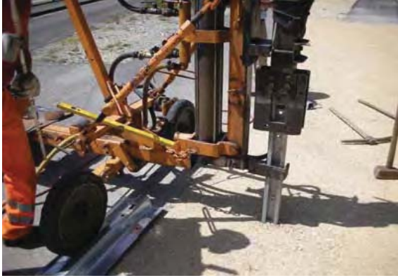
7. Driving posts into ground
