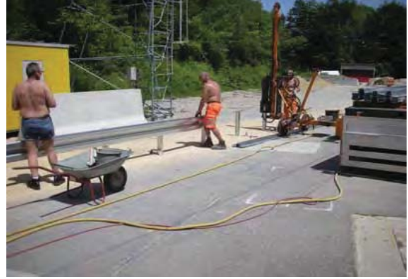
8. Pre Mounting brackets and beams
