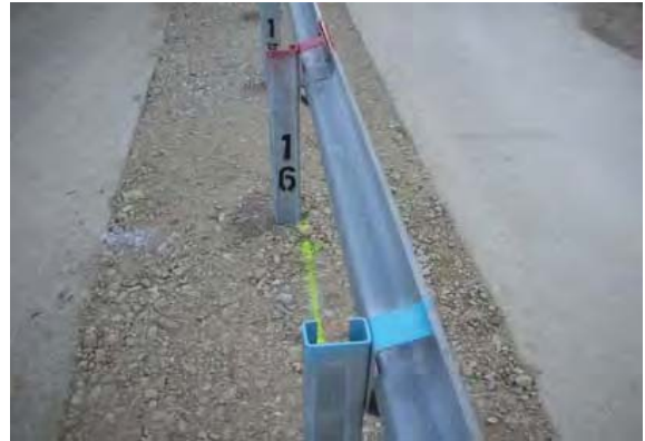
10. completed EASY RAIL
