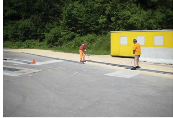
2. Laying out the beams
