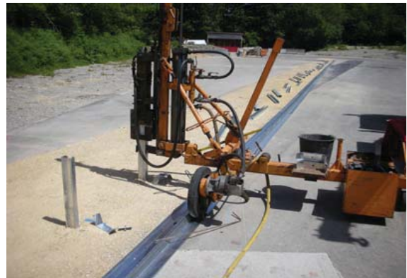
4. ... for piling frame
