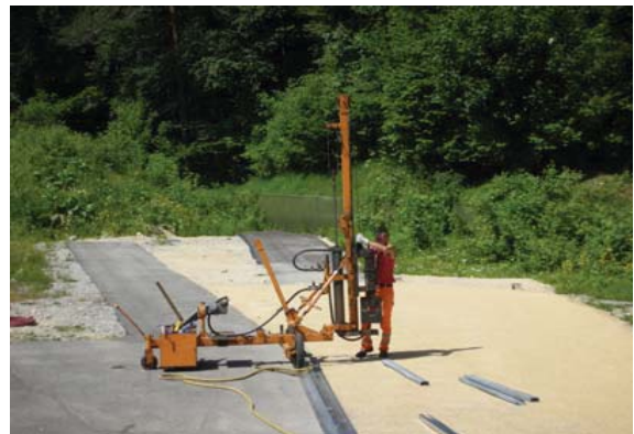
6. Preparing of pile driver
