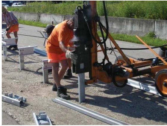
4.9 Rammen der Pfosten Pile driving the posts
