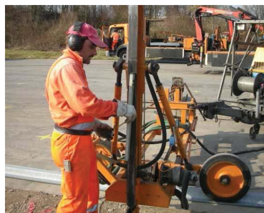
4.8 Lotrechtes ausrichten der Ramme Adjusting the pile driver vertically to the track
