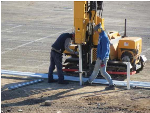
4.7 Lotrechtes ausrichten der Ramme Adjusting the pile driver vertically to the track
