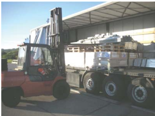
4.1 Abladen des LKW's Unloading the truck
