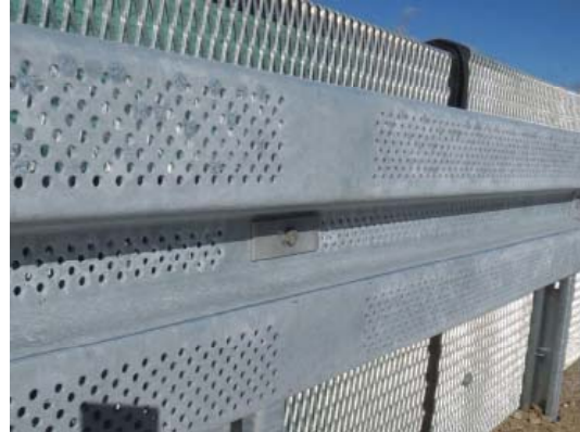
5.4 Verschraubung vorne zwischen Pfosten Front side - fixing between joint
