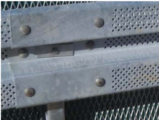
5.3 Verschraubung vorne am SP-Stoß Front side – fixing at beam joint
