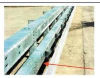
Upper and lower box beams to be mounted withoput any offset!
