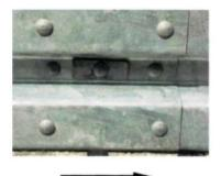
6 pcs. (B-Profile) or 8 pcs. (A-Profile) Bolt, cup head with nib M 16x27, quality 4.6 incl. nut (40.00) and Washer 18(40.30)
