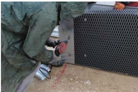
4.9 Montage des End-Deckels am Schallschutzelement f. Übergang (ÜK-SSE) Mounting of the end-cap at the noise absorbing element f. transition (Trans-NAE)
