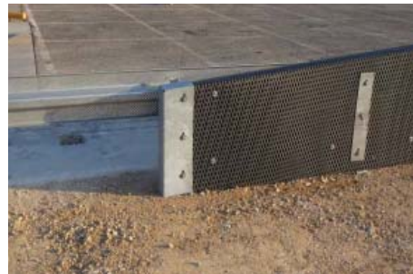
4.9 Montage des End-Deckels am Schallschutzelement f. Übergang (ÜK-SSE) Mounting of the end-cap at the noise absorbing element f. transition (Trans-NAE)
