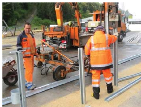
4.9 Rammen der Pfosten Pile driving of the posts
