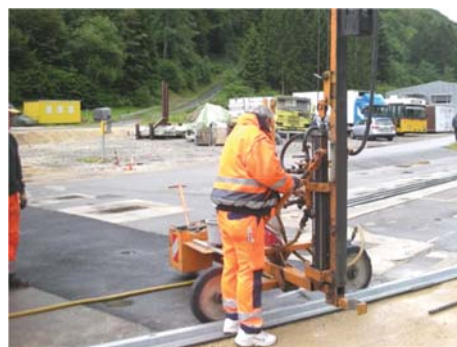
4.8 Lotrechtes ausrichten der Ramme Adjusting pile driver vertically to the track
