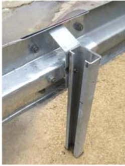
5.1 Detail - EasyRail Bereich Detail - EasyRail section
